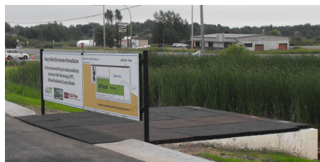
Gravity-feed in-ground vault
