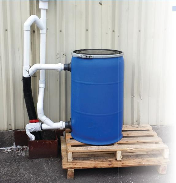
An upflow drum filter used 55-gal drums and peat sorption media to treat storm water runoff at the industrial facility.
